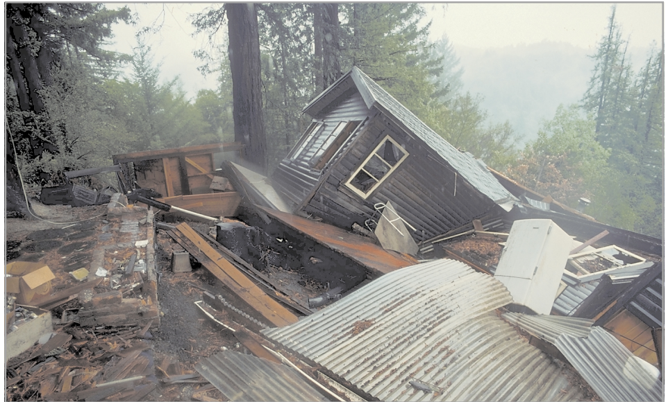
This house in the mountains north of Santa Cruz, California, was destroyed by the October 17, 1989, Loma Prieta earthquake. Shaking was very intense here, close to the epicenter of the magnitude 6.9 shock. However, heavily urbanized San Francisco and Oakland, more than 50 miles to the north, suffered more than 70% of the 63 deaths and the $6 billion to $10 billion in damage caused by the quake.
